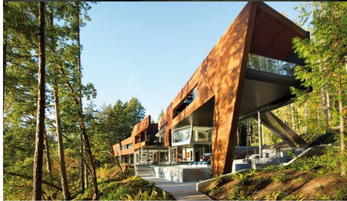
← [71] → [72] Residenza privata Gulf Islands / LUOGO: Vancouver - Canada / PRODOTTO: Medoc / ARCHITETTO: AA Robins / FOTOGRAFO: Ema Peter / ANNO: 2015 © Immagine gentilmente concessa da Ema Peter Photography Private Residence Gulf Islands / PLACE: Vancouver - Canada / PRODUCT: Medoc / ARCHITECT: AA Robins / PHOTOGRAPHER: Ema Peter / YEAR: 2015 © Image kindly authorized by Ema Peter Photography
